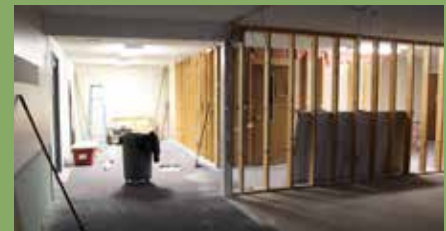
Building a wall to keep the dust and mess under control
