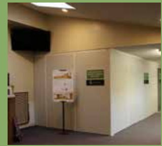
Building a wall to keep the dust and mess under control
